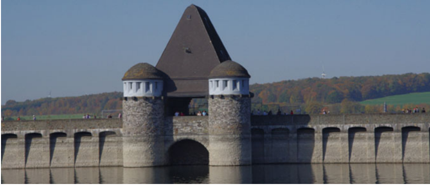
Fig. 1.3 Example of a dam to be monitored (Möhneseedam), © P. Marwedel
